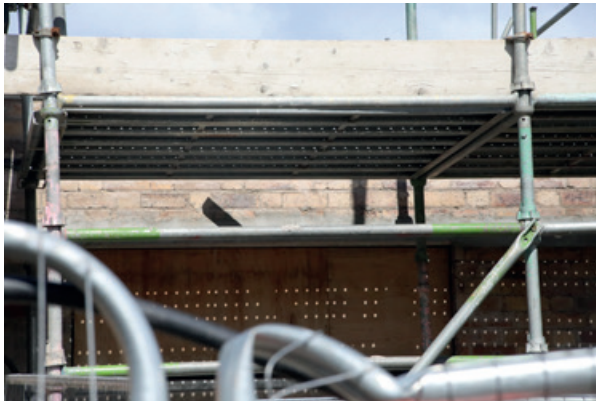
Close-up area where entrance sign is to be applied: existing brick work and concrete.
